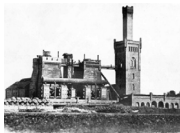
First blast furnace in Ilse, 1861
