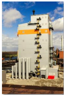
Salzgitter Flachstahl Construction of the pulverized coal injection plant
