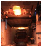
Salzgitter Flachstahl Construction of the RH vacuum degassing plant
